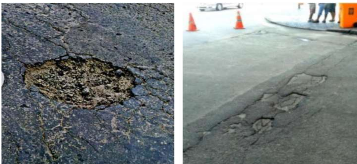
Figura 10 – Painelas / Buraco
