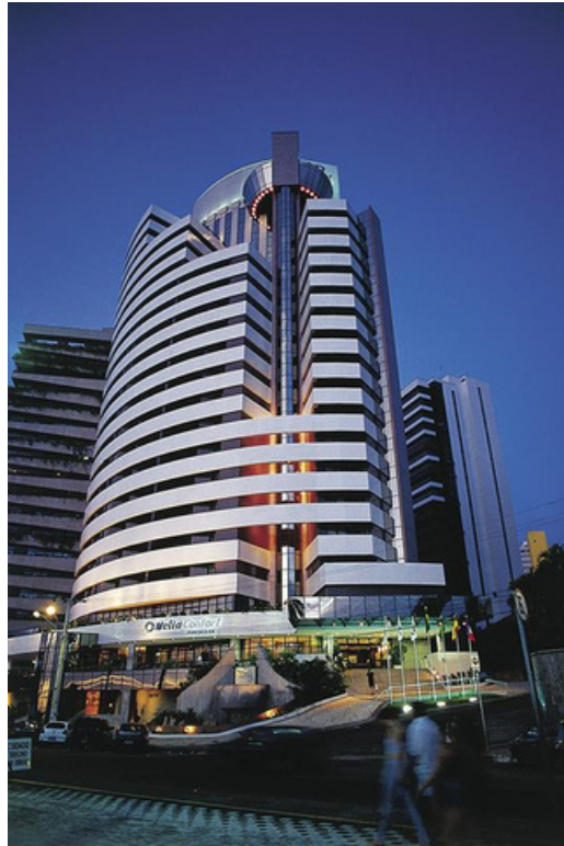
Figura 5 - Fachada Principal – Hotel Meliá Confort
