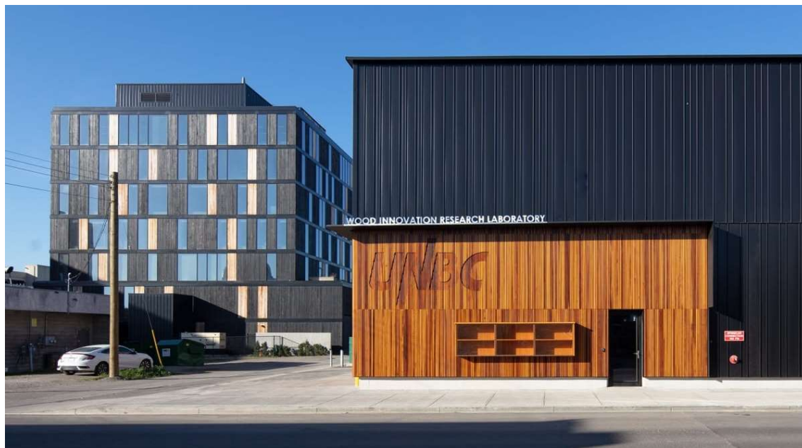
Figura 24: Fachada norte do Wood Innovation Research Laboratory.
